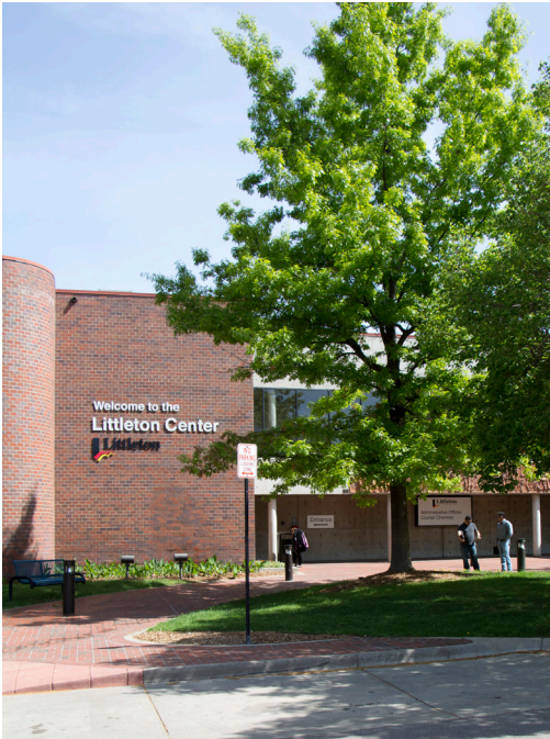
City office building south entrance.
