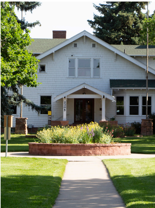
View of paved entry to Geneva Lodge.
