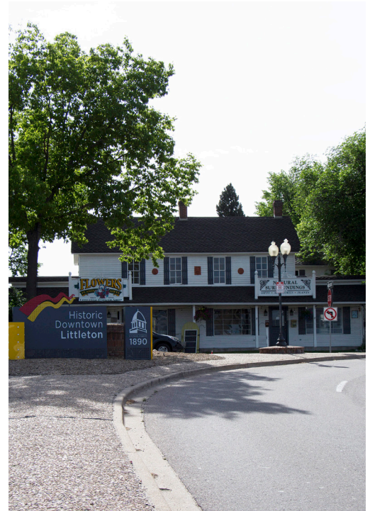
South Santa Fe West entrance to downtown Littleton.
