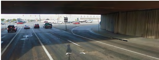
Image 15. Street crossing at Oxford and Santa Fe
