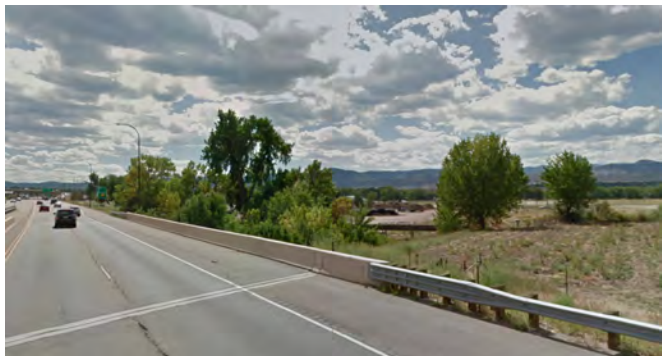
Image 19. Underpass between Mineral and C-470
