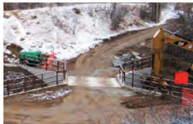
Construction was recently completed on replacement of the Lee Gulch and High Line Canal Trail crossing, east of South Broadway. The new culvert crossing Lee Gulch makes for safer pedestrian, bicycle and equestrian use, replacing a smaller metal
